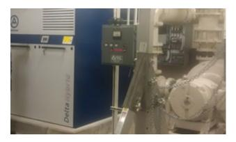
The City of Anacortes replaced a 125HP multistage centrifugal blower (right) with an Aerzen D 62S 75HP hybrid blower (left).
