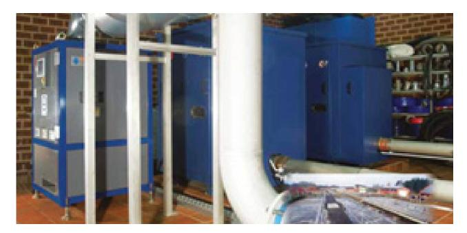
Figure 1 Aerzen AT turbo blower and two PD blowers processing air at a Bremervörde, Germany WWTP.
